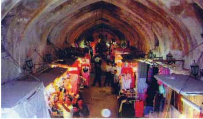
The Historic Covered Bazaar in Kirkuk (Kayserrîye Bazaar)
