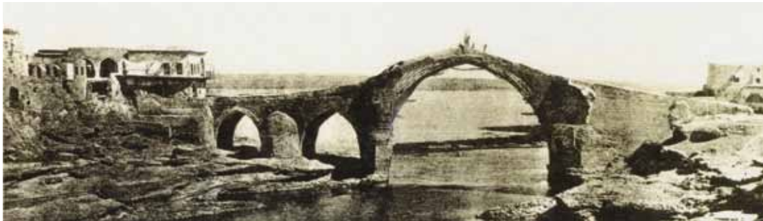
The Altinköprü Nâhiye – The oldest photograph of the Great Bridge
