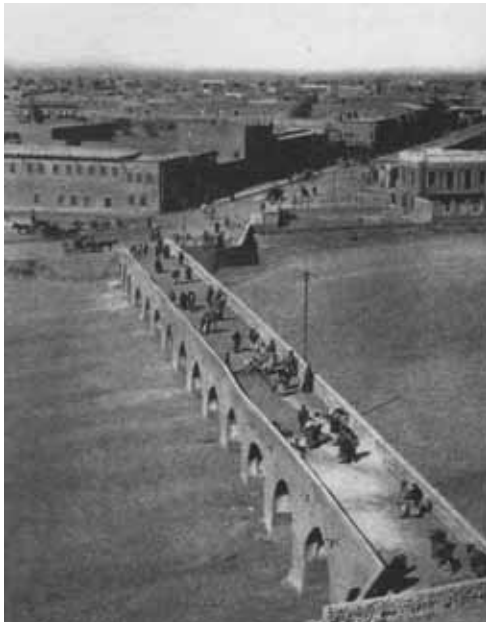
Muşir Nafiz Pasha's stone bridge with sixteen arches over the Hassa Creek
