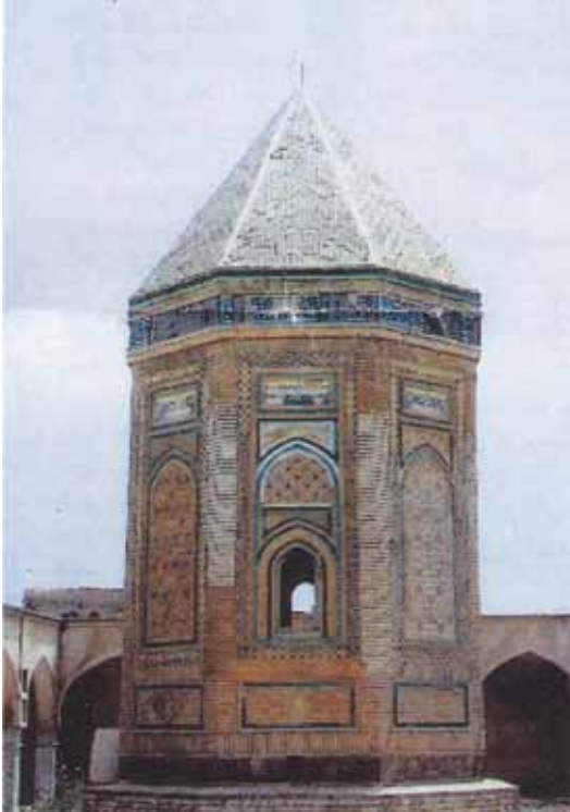
Fortress and its Inscription (It has an octagonal shape and is 10 meters tall).
